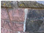
The primary foundation walls on the original structure are eight-face stone laid in an "Ashlar" pattern. In general, the masonry foundation walls are in fair to good condition, isolated areas, however, are showing signs of settling and cracking. These areas include several spalling stones, visible cracks, and areas of deteriorated or inappropriate mortar.
