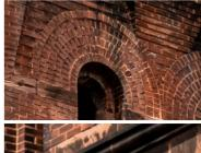
The steeple is constructed primarily of brick masonry with stone banding. The general condition of the masonry appears consistent with the condition of masonry on the primary church building, with some areas/elements in need of repair or reconstruction.
