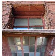
Some of the masonry opening headers (in particular on the school wing addition) are supported by steel bearing lintels - angles and plates. These are subject to deterioration and rusting due to exposure to moisture.
