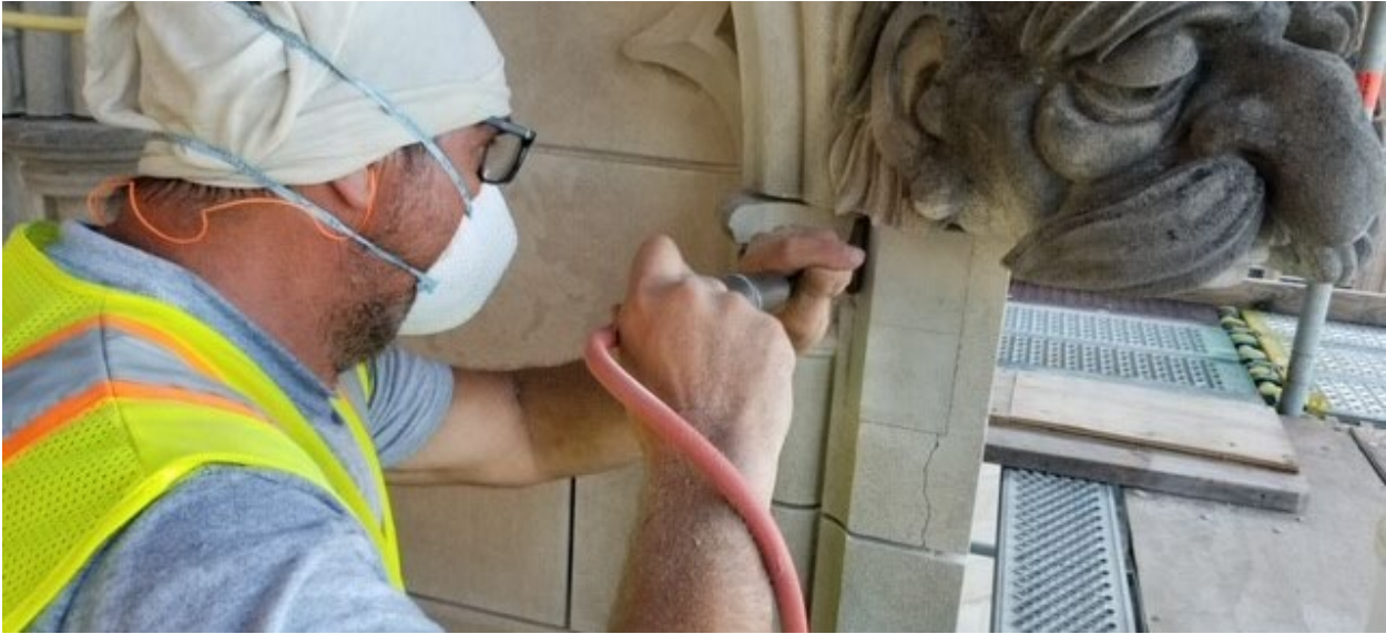
Lorton Stone repairing a damaged gablet on the Washington National Cathedral Washington, DC. Photo by Joe Alonso.
