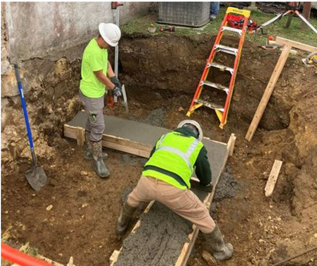
Woodruff Construction forming the footings for the emergency egress stairs at Amana Church Society Middle Amana, IA
