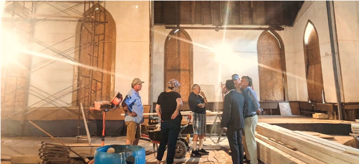
Executive Director Robert Leath and EHC Treasurer Tom Credle meeting with Edenton Town Manager Corey Gooden, Project Architect Laurie Jackson, and Construction Manager Don Faircloth to review the progress of the structural stabilization at Kadesh AME Zion Edenton, NC. Photo by Alexis Tobias-Jacavone.
