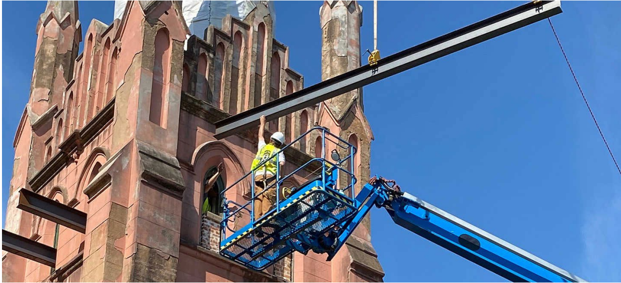
Temporary steel beams being installed at Trinity Episcopal Church Abbeville, SC. Photo by Preservation South Carolina.
