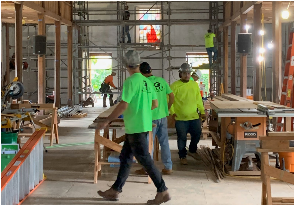
Ali'i Builders installing steel beams in Mokuaukaia Church Kailua-Kona, HI
