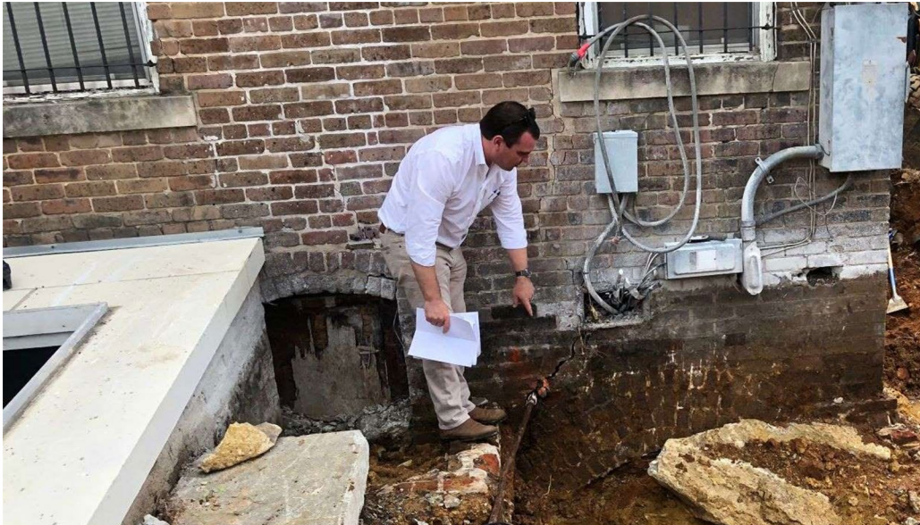
ArchitectWorks assessing the condition of the foundation at 16th Street Baptist Church Parsonage Birmingham, AL
