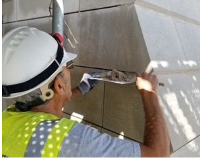
Left: Lorton Stone repointing mortar joints on the Washington National Cathedral, Washington, DC. Photo by Joe Alonso. Center: Completed mortar repointing between the decorative terra cotta band and brick at the First Baptist Church of Asheville, NC. Photo by WxProofing. Right: Restored grotesque on Saint Mary of the Immaculate Conception Catholic Church, Indianapolis, IN. Photo by Rosemary Dorsa.
