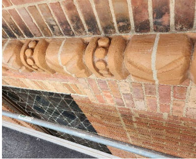
Left: Lorton Stone repointing mortar joints on the Washington National Cathedral, Washington, DC. Photo by Joe Alonso. Center: Completed mortar repointing between the decorative terra cotta band and brick at the First Baptist Church of Asheville, NC. Photo by WxProofing. Right: Restored grotesque on Saint Mary of the Immaculate Conception Catholic Church, Indianapolis, IN. Photo by Rosemary Dorsa.
